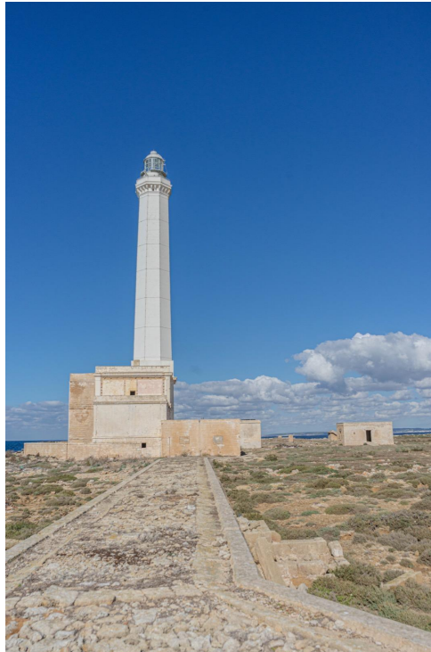
Fig 4. Lighthouse on Sant'Andrea Island, built in 1866. Source: Photograph by Alfredo Giungato.
